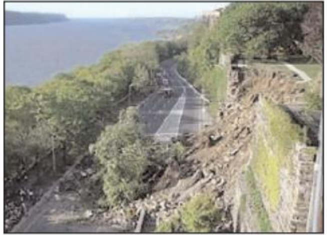
Retaining wall collapse on May 12, 2005
